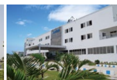
Delta Rudrapur LEED-India Gold
